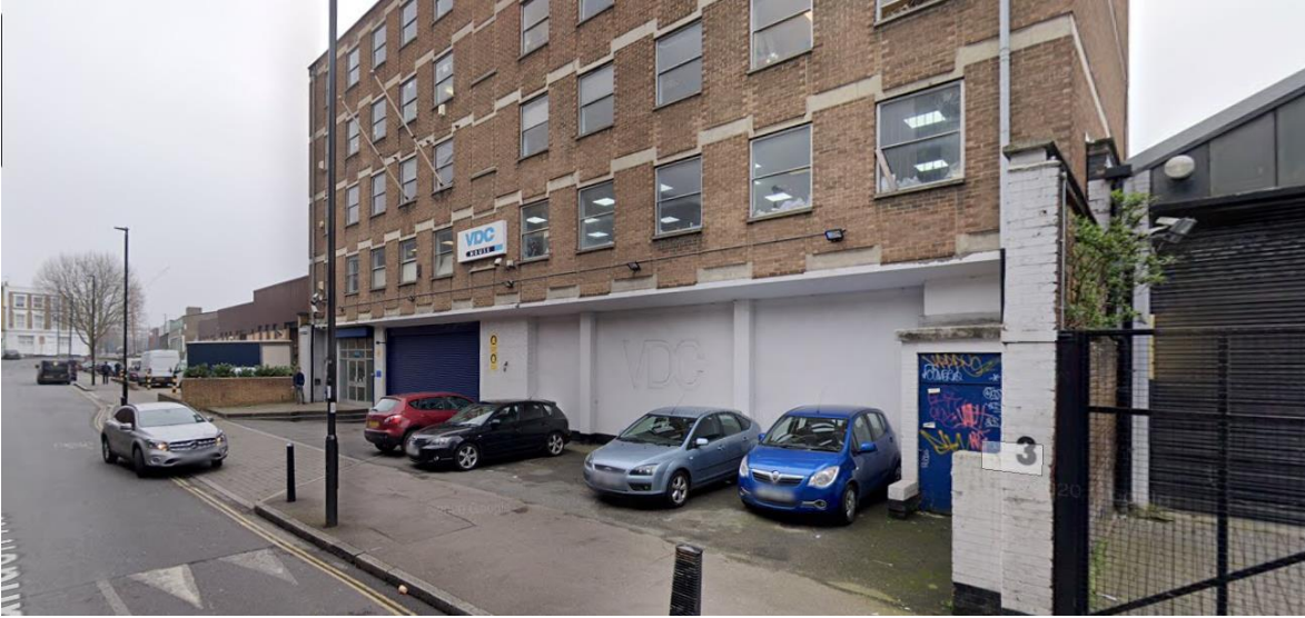
Fig. 10.10: Front of existing Site
