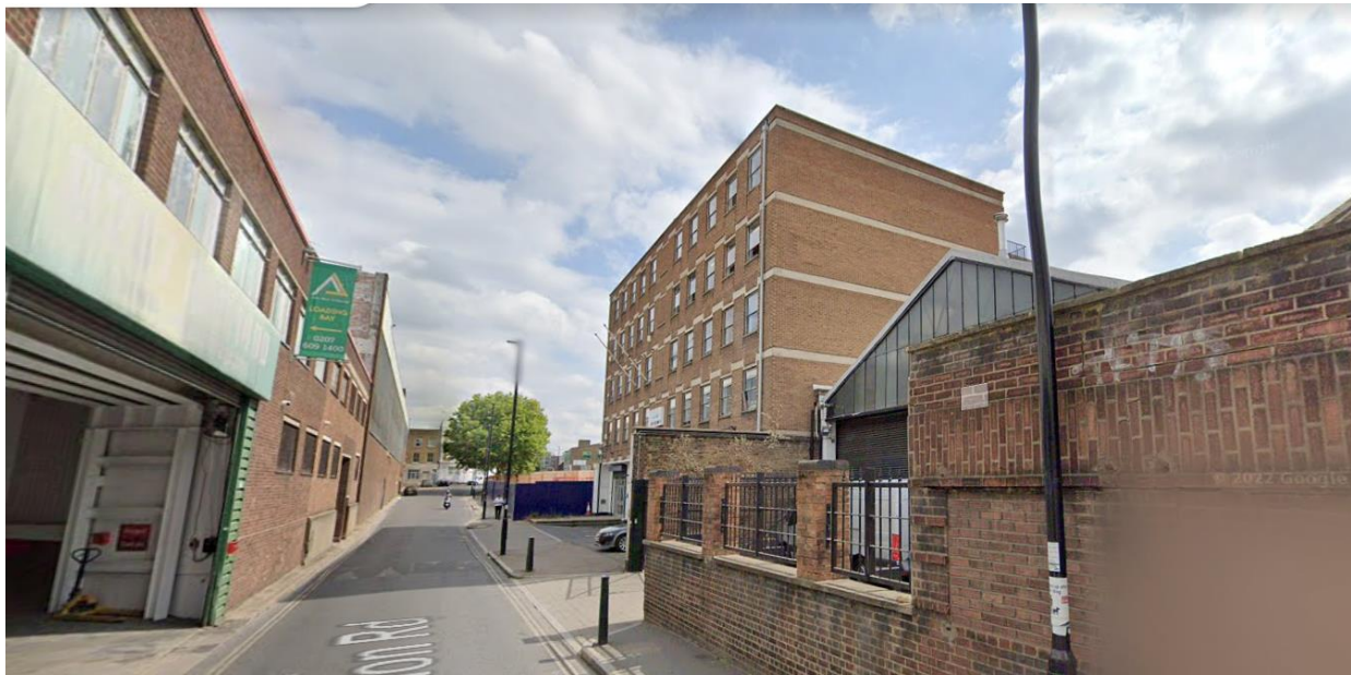
Image 3.4: Looking east from the junction with York Way showing front elevation
